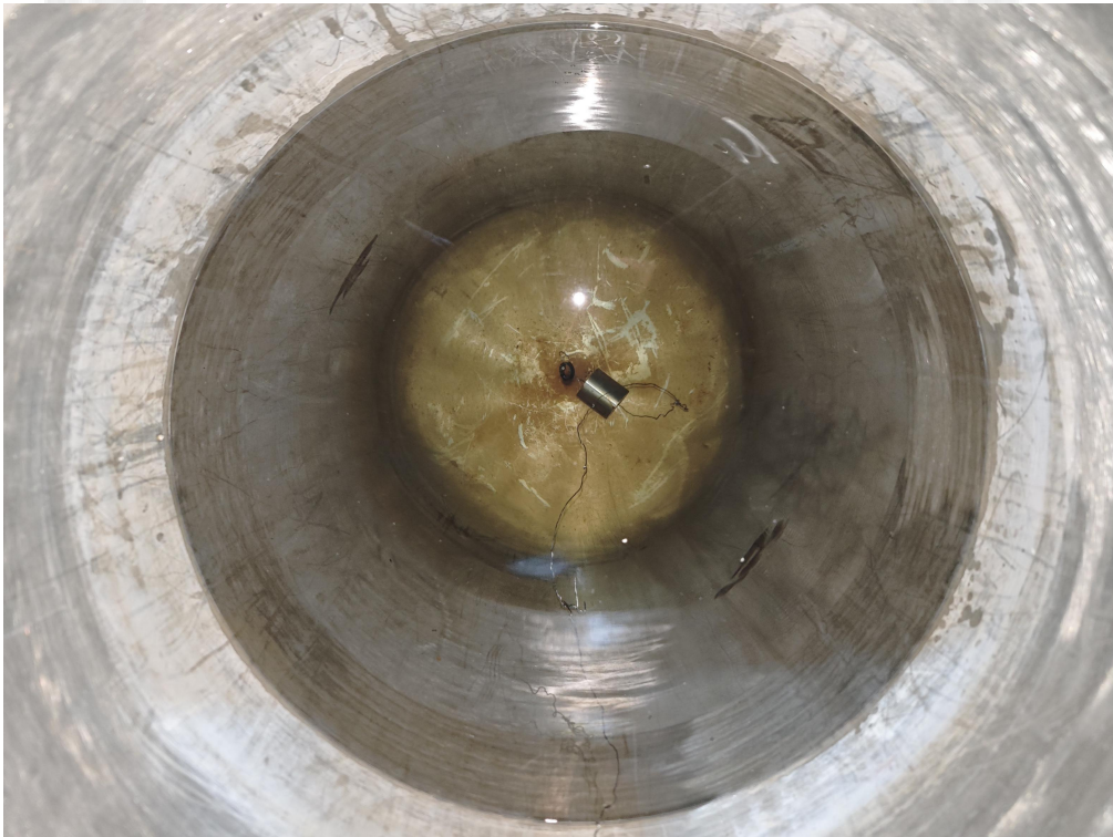
Photo 6 Before test view
